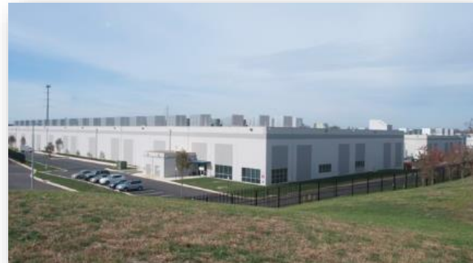
AWS Datacenter – New Albany, OH
