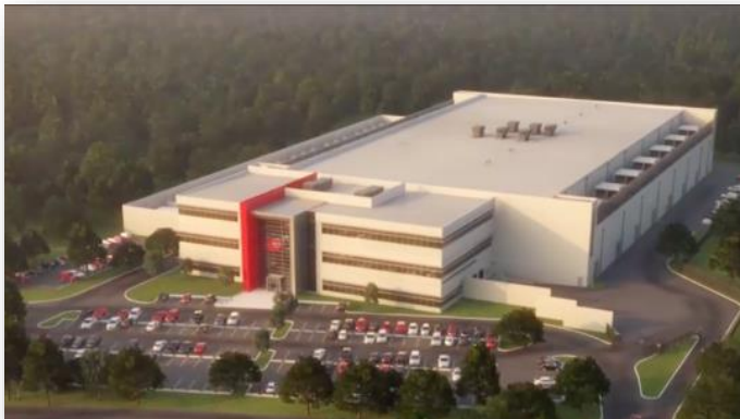
QTS Datacenter – Ashburn, VA
