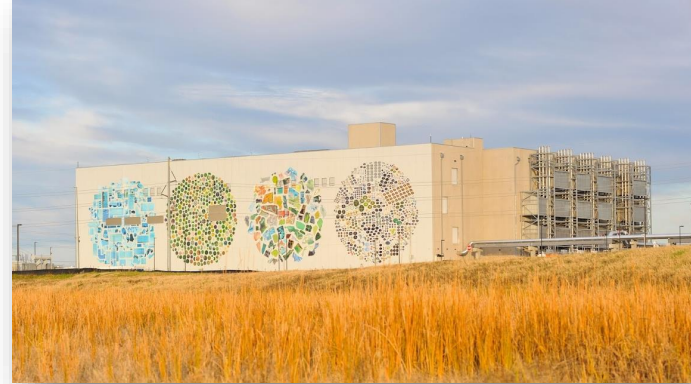
Google Datacenter – Mayes County, OK
